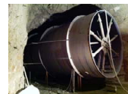
Steel liner with spider bracing system
